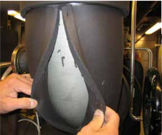
The way it should be: suitable, correctly dimensioned insulation materials prevent condensation
