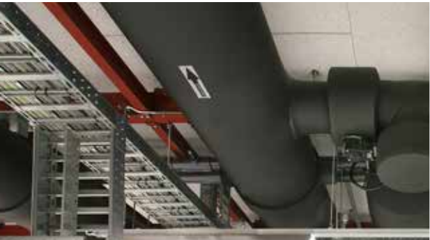
The way it should be: suitable, correctly dimensioned insulation materials prevent condensation
