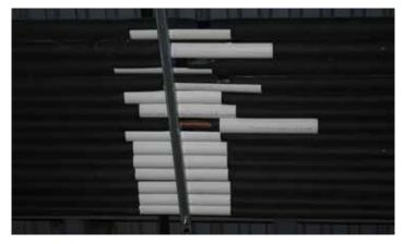
With standard metal or plastic supports, insulation tearoff occurs with pipe saddle displacement and exposes critical lines to the effects of friction.
