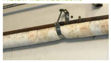
Insulation compression at suspension locations breaks the thermal barrier. This results in thermal bridging and could cause condensation, freezing points and mold growth.
