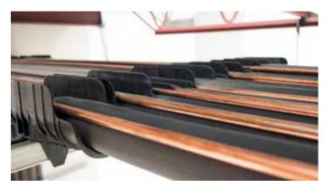
Insuguard saddles have high walls which protect the liquid lines from strut, threaded rod and hangers and carry the weight of the pipe without thermal bridging.
