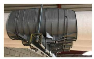
Insuguard's revolutionary curved edge saddle design allows the insulated pipe to expand and vibrate within the support with no possibility of tear-off.
