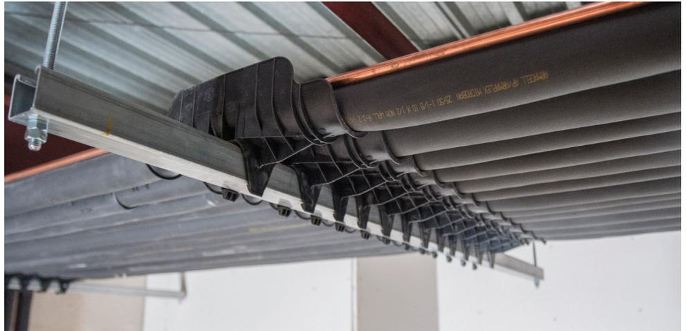
Potential issues with pipe suspension or mounting systems include shifting/falling saddles, condensation and mold growth, freezing and thawing, refrigerant leaks, insulation tear-off, and inefficient labor and material use. With normal pipe movement and expansion, saddles can slip out of place, exposing the insulation to pressure and compression. For cold systems, thermal bridging
